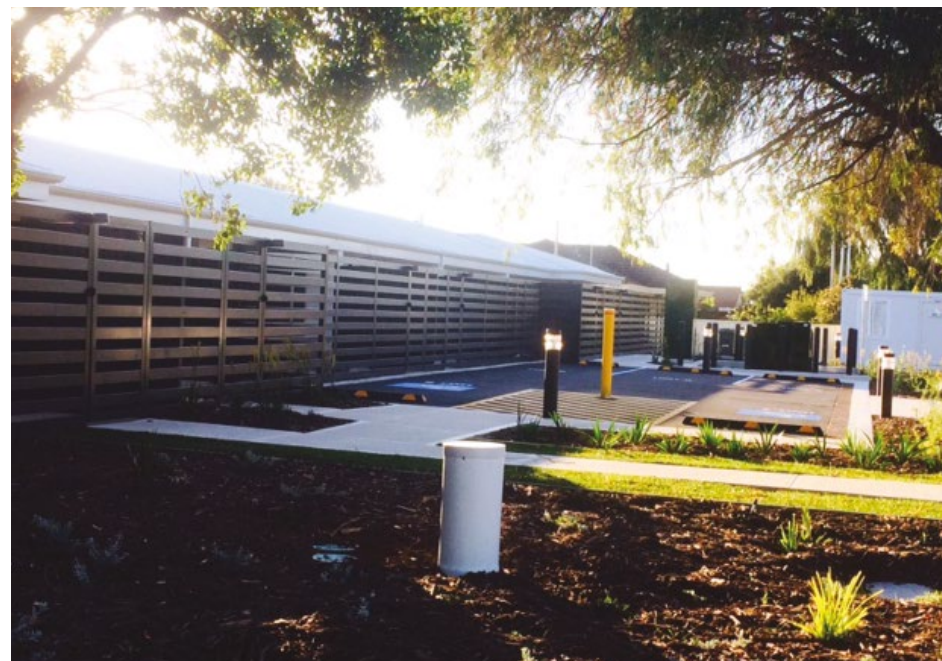
Rockingham step-up, step-down service – anticipated to be operational by November 2016
