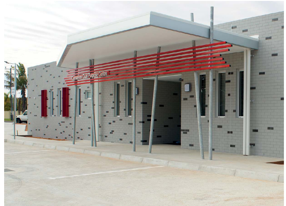
Carnarvon Dual Purpose Centre (Sobering Up Centre) PHOTO COURTESY OF SANDOVER PINDER ARCHITECTS
